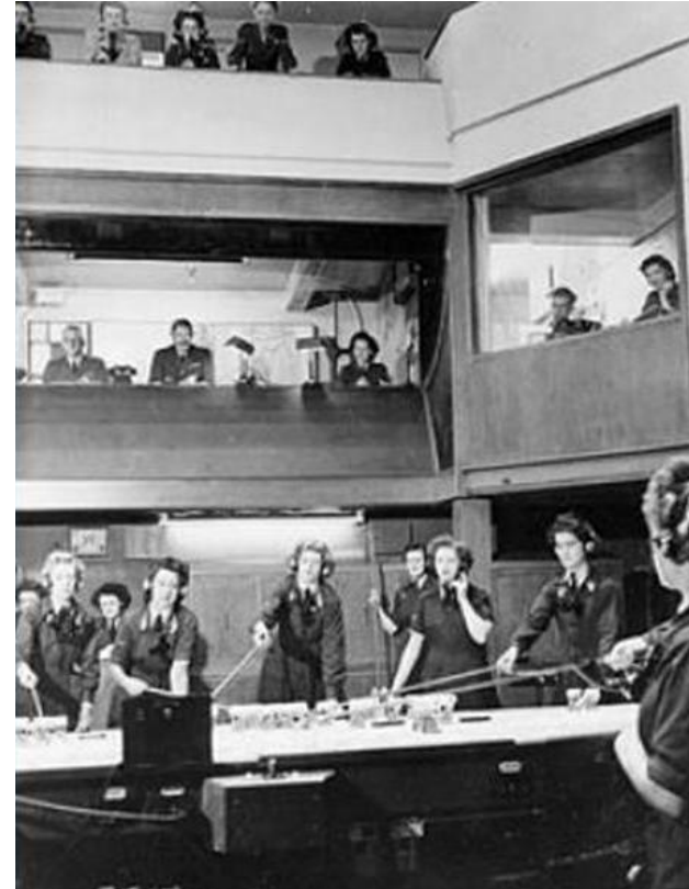
Operation Room at Air Group 10
