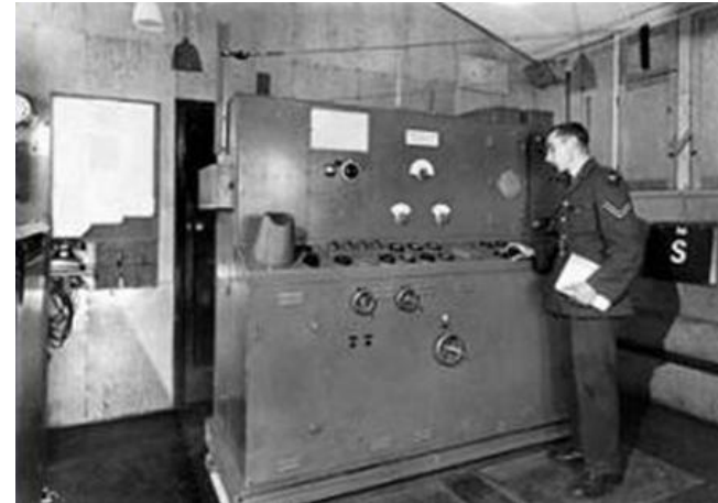
Chain Home Low Transmitter
