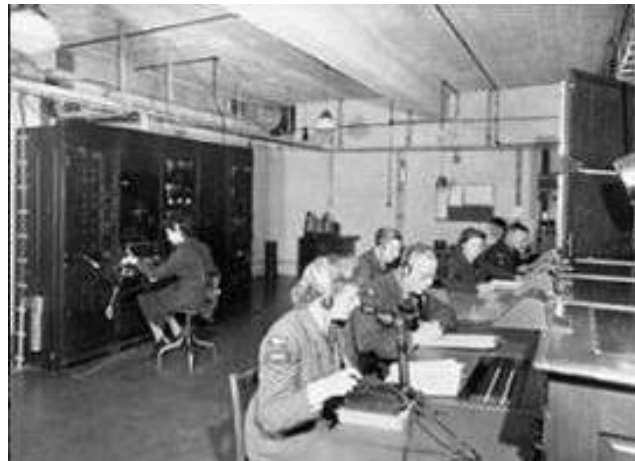
Chain Home Receiver Hut
